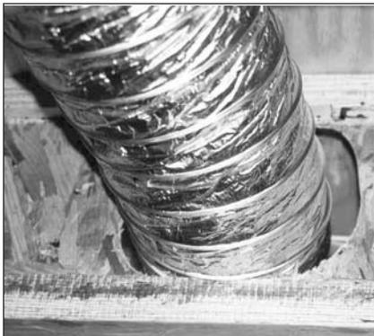
Incredible, but true. There is no resistance in this joist. To be replaced at the expense of the contractor.
